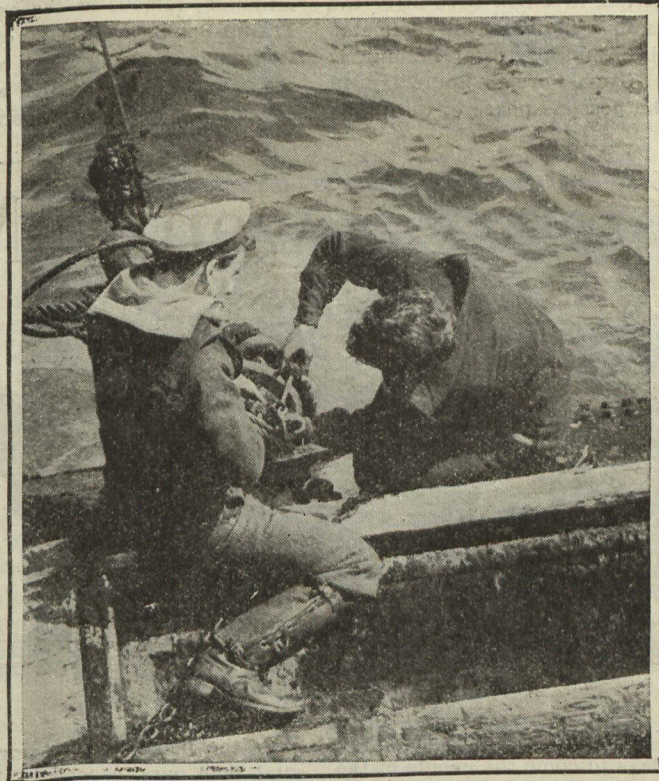
Marine Outpost laying Nets from Drifters to catch U-Boats.
