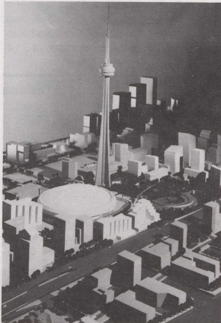
Model of domed stadium with largest retractable roof to be built next to the CN Tower in Toronto, Ontario.
