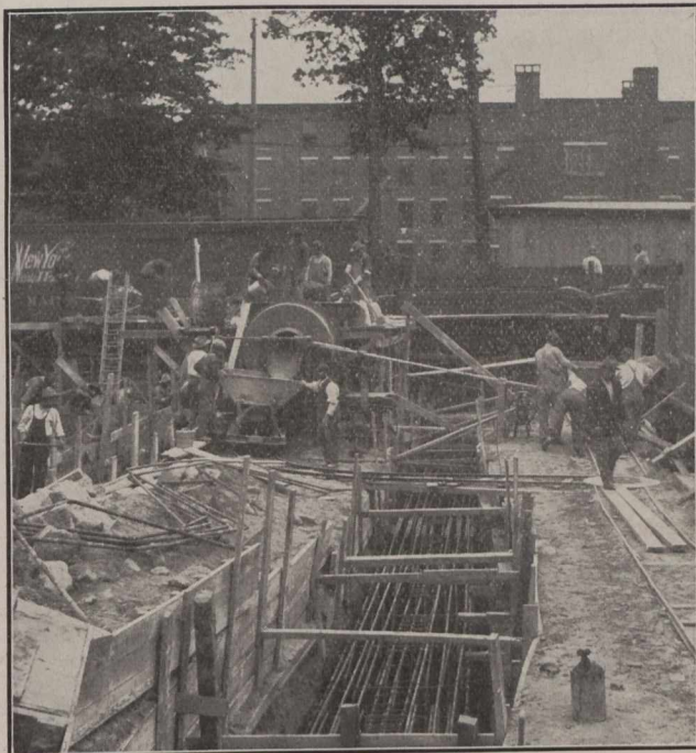
Reinforcement in Place.
