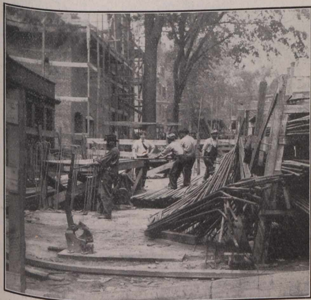
Shaping Reinforcement.
