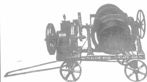
The Wetlauer Concrete Mixer is especially adapted for all Farm Concrete Work—Brick, Block, Barn Floors, Foundations and Silo building. The Wetlauer Concrete Mixer mixes quickly and thoroughly, and Government test has proven that it makes a concrete that is absolutely impossible to make by hand. This Mixer will save you money on your own Cement work and You Can Earn Money by doing work for your neighbors.
