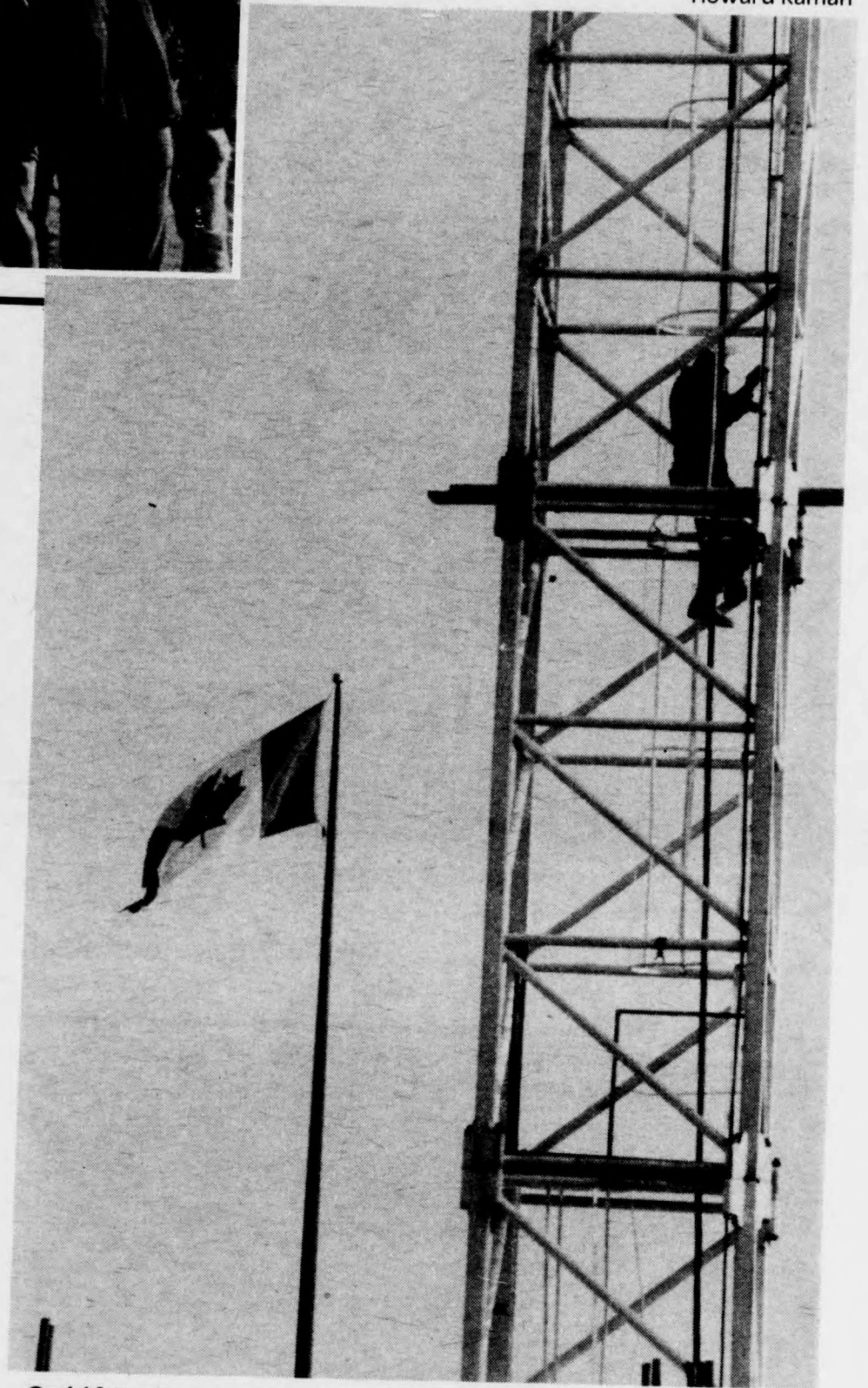
Getting to work on the entry pavillion
