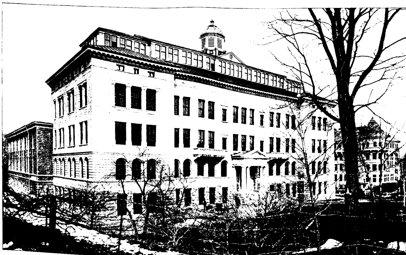
WM. WORKMAN WORKSHOPS AND LABORATORIES.
