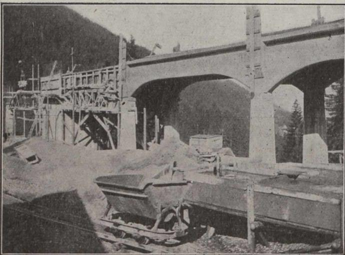
Fig. 3.—Long Span Continuous Girders of Approach.
