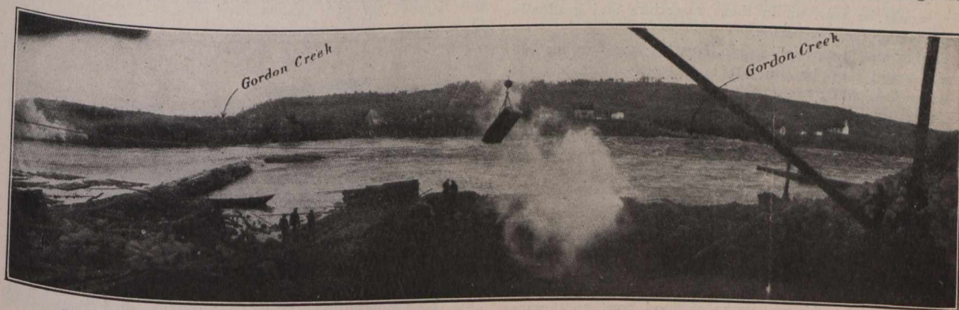
Fig. 1.—Timiskaming Dam, November, 1910. Coffier Dams, Quebec Channel, Stopped by Autumn Floods.
