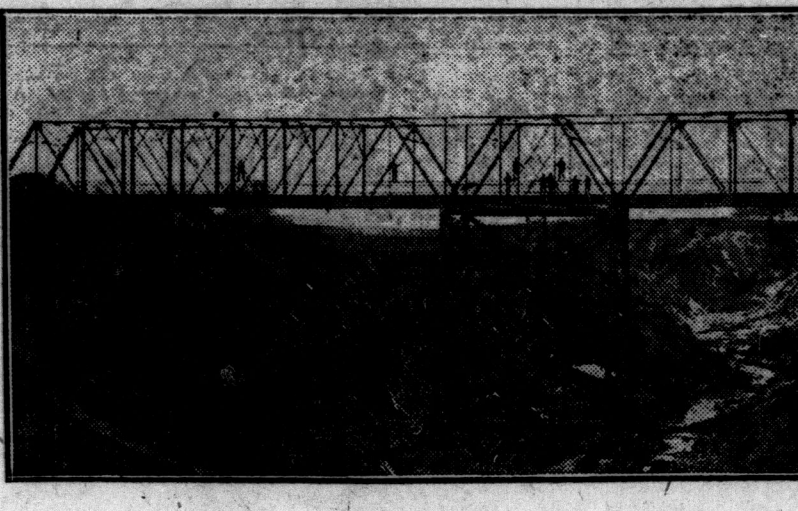
NEW BRIDGE OVER STALTER GULLY. Gully, in the township of Malahide, bridge is one of the finest of its kind and is now open to traffic. The bridge has just been completed over Stalter.
