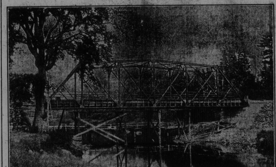
THE NEW BRIDGE AT ARMSTRONG'S CORNER. Sub-structure consists of two concrete U abutments 25 feet in height, resting on a hard pan of gravel below the surface. The superstructure consists of a fixed through riveted steel span of 94 feet, with a reinforced concrete river bed surface, with approaches of stone and earth. The road way, gutter and side curb, wearing surface of the roadway being an asphalt McAdam. This bridge is the last word in permanency of construction for a bridge of this class.
