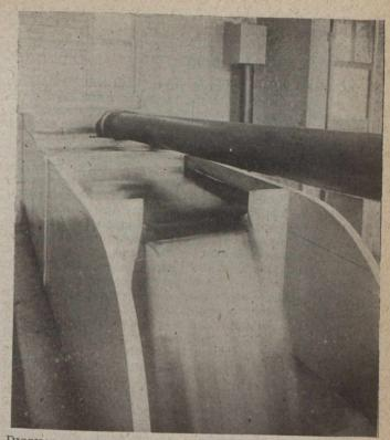
DISCHARGE INTO WEIR BOX OVER CONCRETE STORAGE BASIN AT GALESBURG, ILL.
