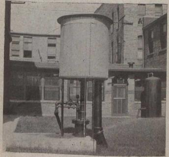
WELL-HEAD AND SEPARATING TANK AT GALESBURG, ILL.—AIR RECEIVER AT THE RIGHT
