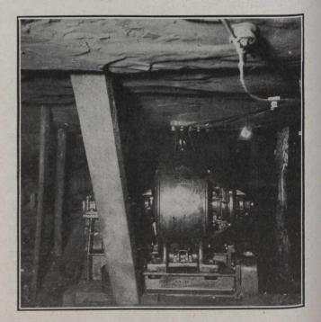
Heretofore, while it has been possible under some conditions to start them from the power house, most motors driving nine pumps and fans had to be started by hand. Hence, if the power went off temporarily for any reason, the motors stopped, necessitating an attendant to go to each station to start them again.
