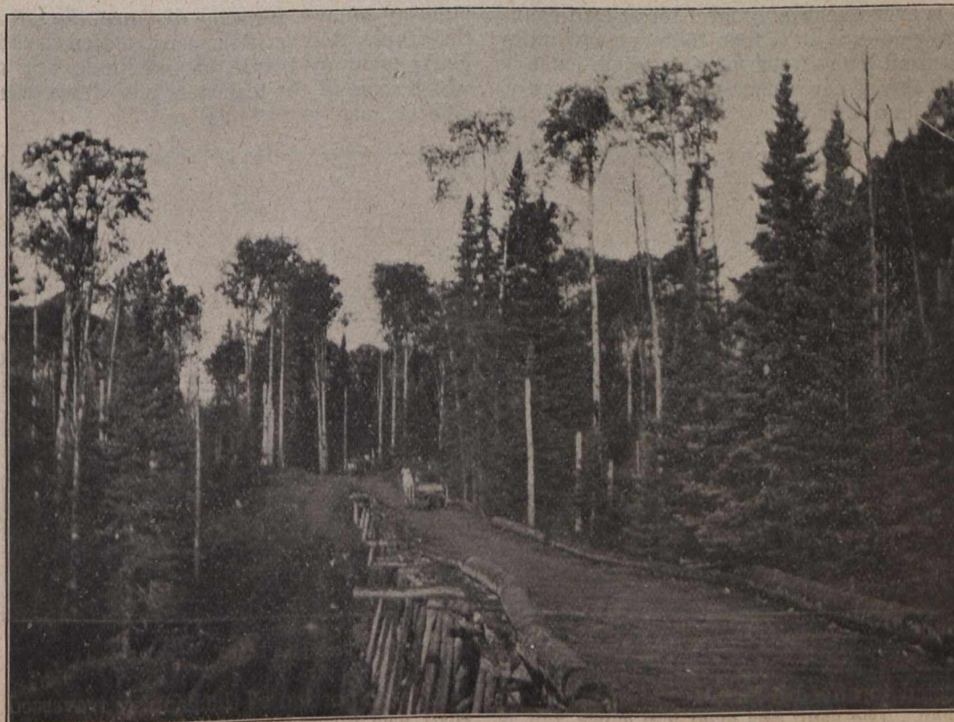
On The Kelso Road. Showing Old Trestle Built by Tie Contractors and Now Used as Highway Bridge.
