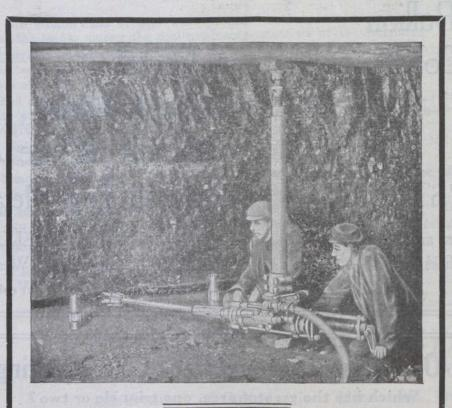
200 "47" Radial Coal-Cutters are in use in one mine in Eastern Canada—the average cost of repair has been found by the Company's own officials to be \$1.35 per month.
