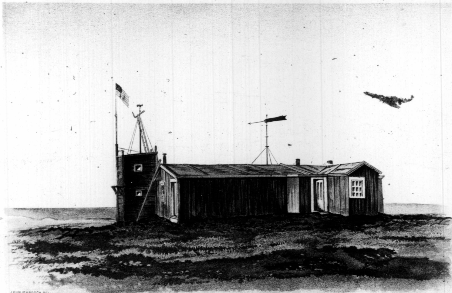
FRONT VIEW OF MAIN BUILDING, UNITED STATES SIGNAL STATION, POINT BARROW, ALASKA.
