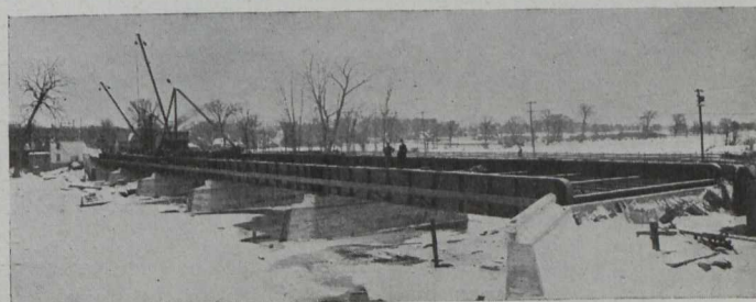
View of Abutments, Piers and Superstructure Partly Completed.
