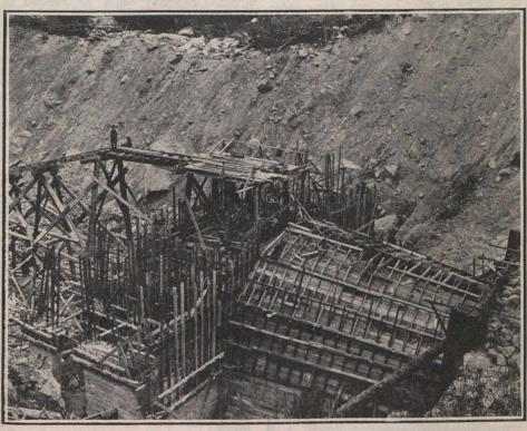
Connaught Tunnel, C.P.R., side view of forms for construction of portal and ventilator nozzle.
