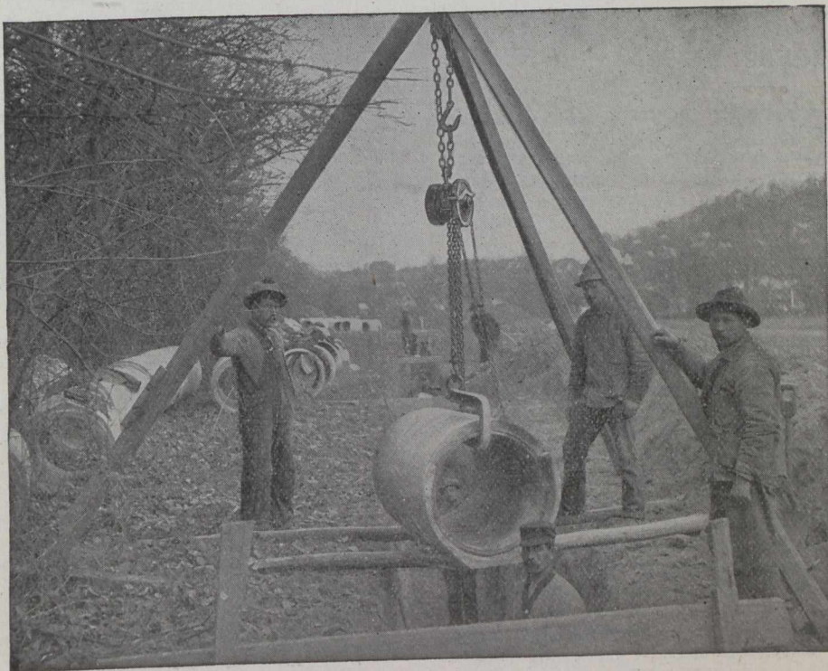
A Triples Block hung from a temporary rigging and used for laying pipe.
