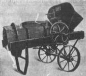
Street Work, and all classes of concrete work where a thorough mixture with but small capacity is required.
