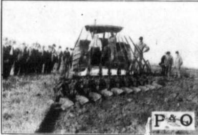
Whenever you see an Engine Gang Plow with the levers pointing to the centre of the platform, it is a P. & O. Mogul. It is exclusive. No other plow is constructed in this way and it thus becomes an easily seen distinguishing mark of the greatest and most easily operated gang plow in the market.
