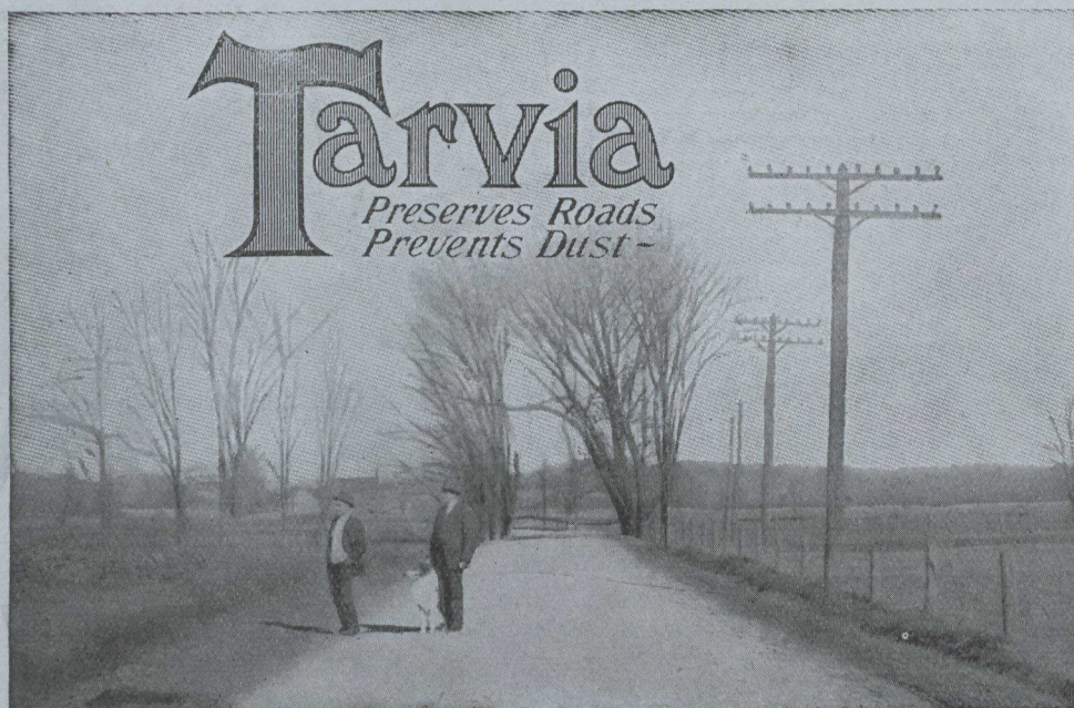
Sherbrooke-Derby Line Highway, (Provincial Government) Near Lenoxville, Quebec. 7 miles of Tarvia Filled Macadam—Penetration Method
