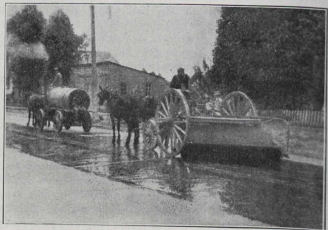
Sprinkling and Spreading Bitumen
