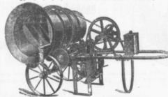
These machines are made to mix either continuously or in be operated either by Hand Steam or Gasoline Power.
