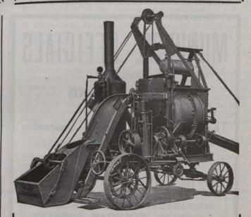
LONDON PAVING MIXER. A forward Loader and rear discharge. No wheelbarrows required. One-third labor saved. The delivery spout is 18 ft. long, swings in a complete circle, distributing the concrete to any part of the roadway. Cuts down the cost. Produces better concrete.
