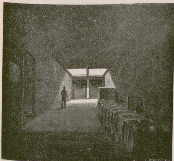
BASEMENT FITTED WITH ORDINARY SIDEWALK LIGHTS.
