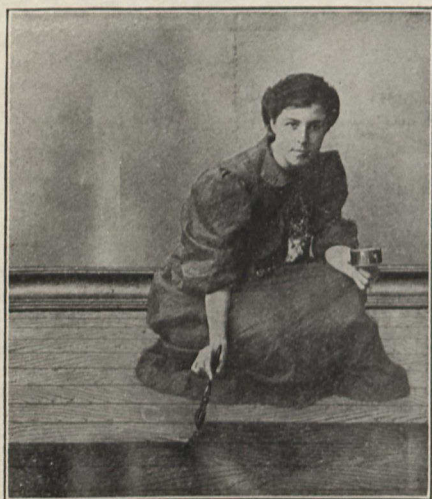
Floorglaze is the only Perfect Floor Finish
