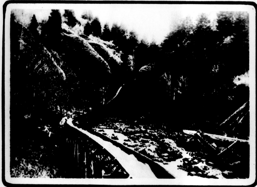
In the Oregon forests, the lumbermen shoot logs down this flume at the rate of four miles in twelve minutes
