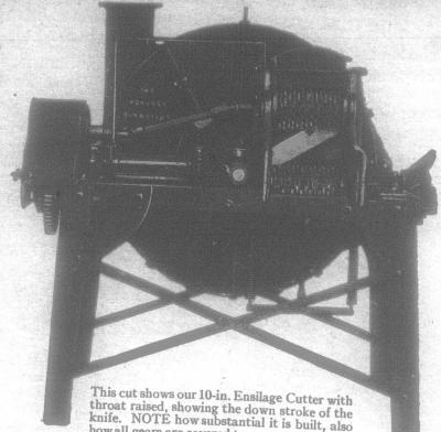
throat raised, showing the down stroke of the knife. NOTE how substantial it is built, also how all gears are covered to prevent accidents.
