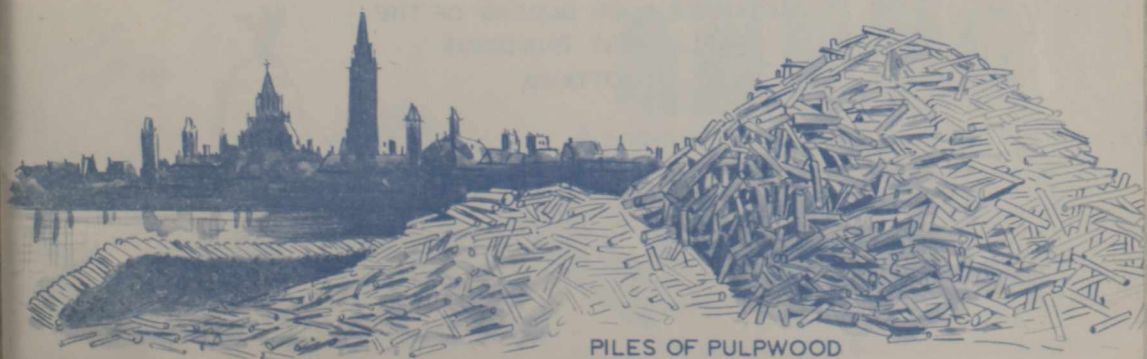
PILES OF PULPWOOD
