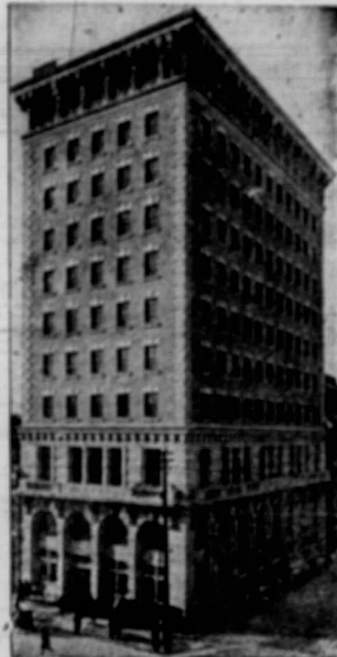
Union Bank Building, Winnipeg
