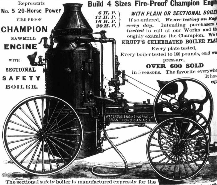
The sectional safety boiler is manufactured expressly for the "North West" trade. This boiler is so arranged that it is readily taken apart in section enabling purchasers to clean thoroughly every part of it and prevent burning out. We know from experience this is absolutely necessary with the alkaline waters of the great Western prairies. Largely used by the Pacific Railway Company and all the large Colonization and Rancho Companies.
