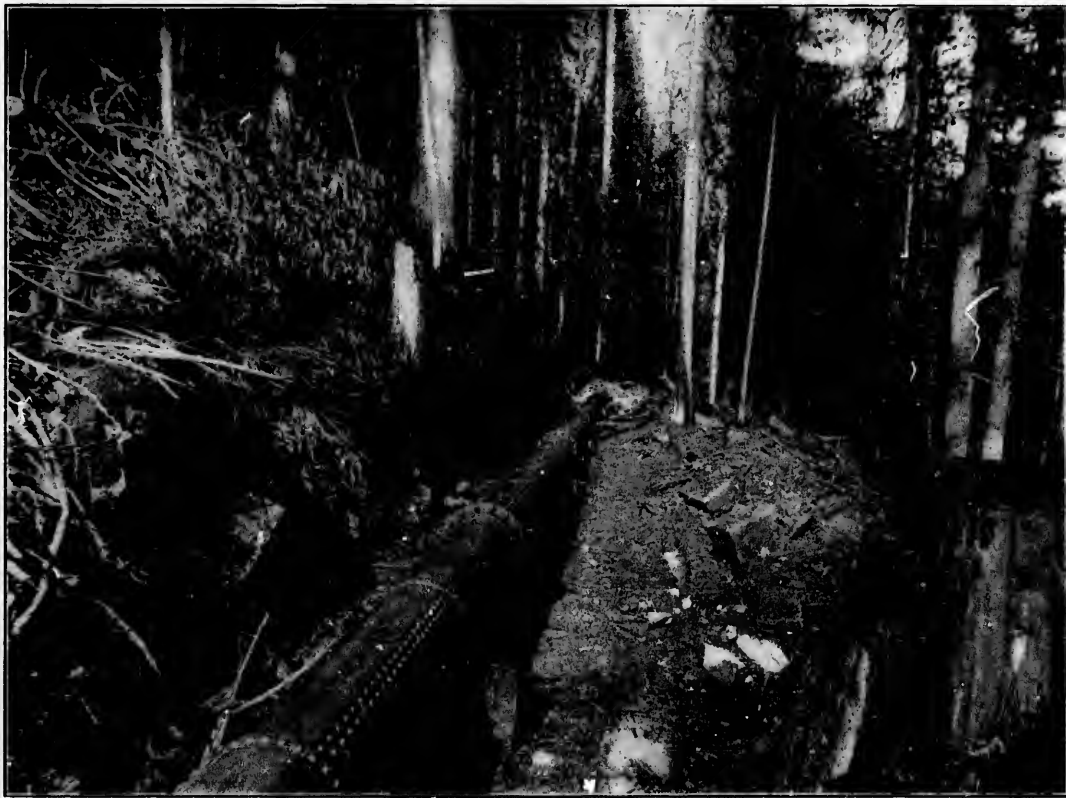
FLANGED STEEL HIGH PRESSURE PIPE LINE, TOTAL LENGTH 7000 FT.
