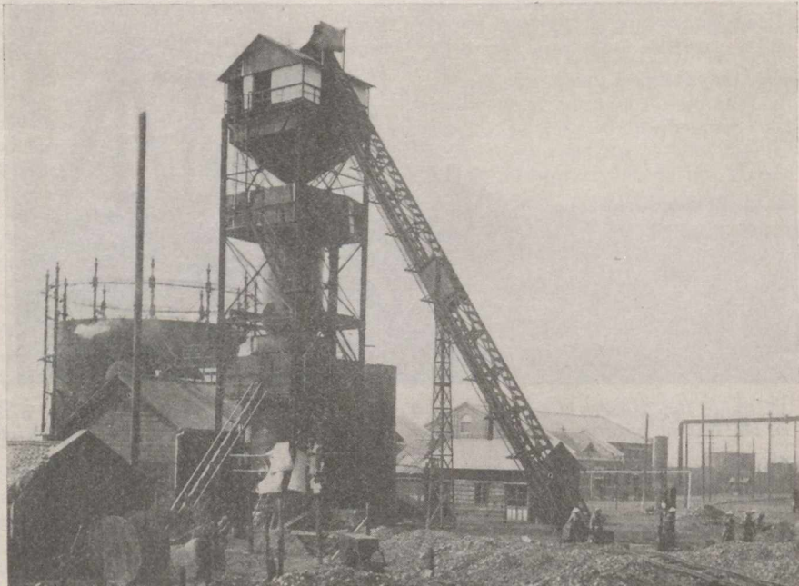
Fig. 15 shows a full-sized testing plant for extracting oil from the shale that covers the coal at Fushun Colliery
