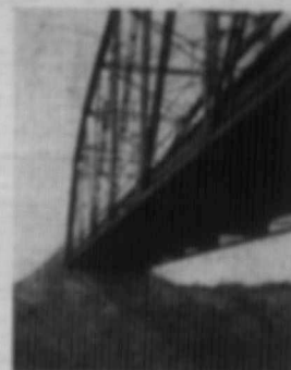
A 150-ft. Steel Span on Re-inforced Concrete Abutments
