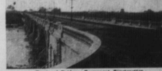
Types of Bridges, Permanent Construction Upper scene: 104-ft. steel span on re-inforced concrete abutments; lower three scenes: the 10-arch, re-inforced concrete bridge at Saskatoon, showing view from down stream, the longest arch (span 150 feet, roadbed 70 feet above water) and at the bottom: the roadway.
