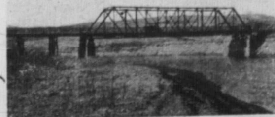
Types of Bridges, Semi-Permanent Construction From top to bottom: Typical single span pile bridge; multiple span pile bridge; multiple span pile bridge with ice breakers; composite bridge with wooden approach spans to steel span on pile piers.
