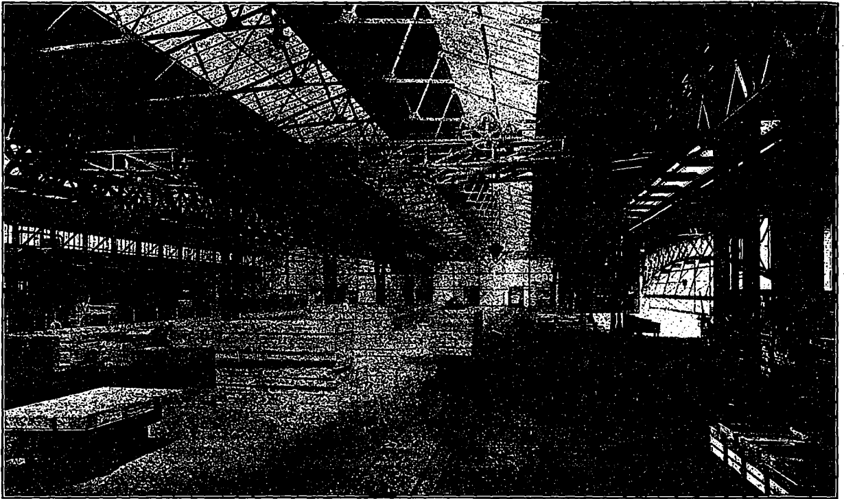
View of Packing and Shipping-Room for galvanized sheets of the plant of John Lysaght, Limited, at Bristol, Eng.
