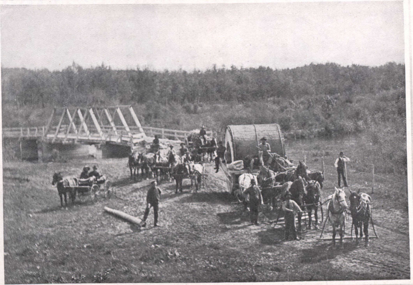
A Marine Boiler made into a "Roller" and "Rolled" a Hundred Miles, from Edmonton to Athabasca Landing.
