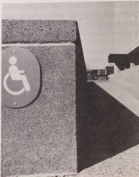
Ramps for building accessibility.
