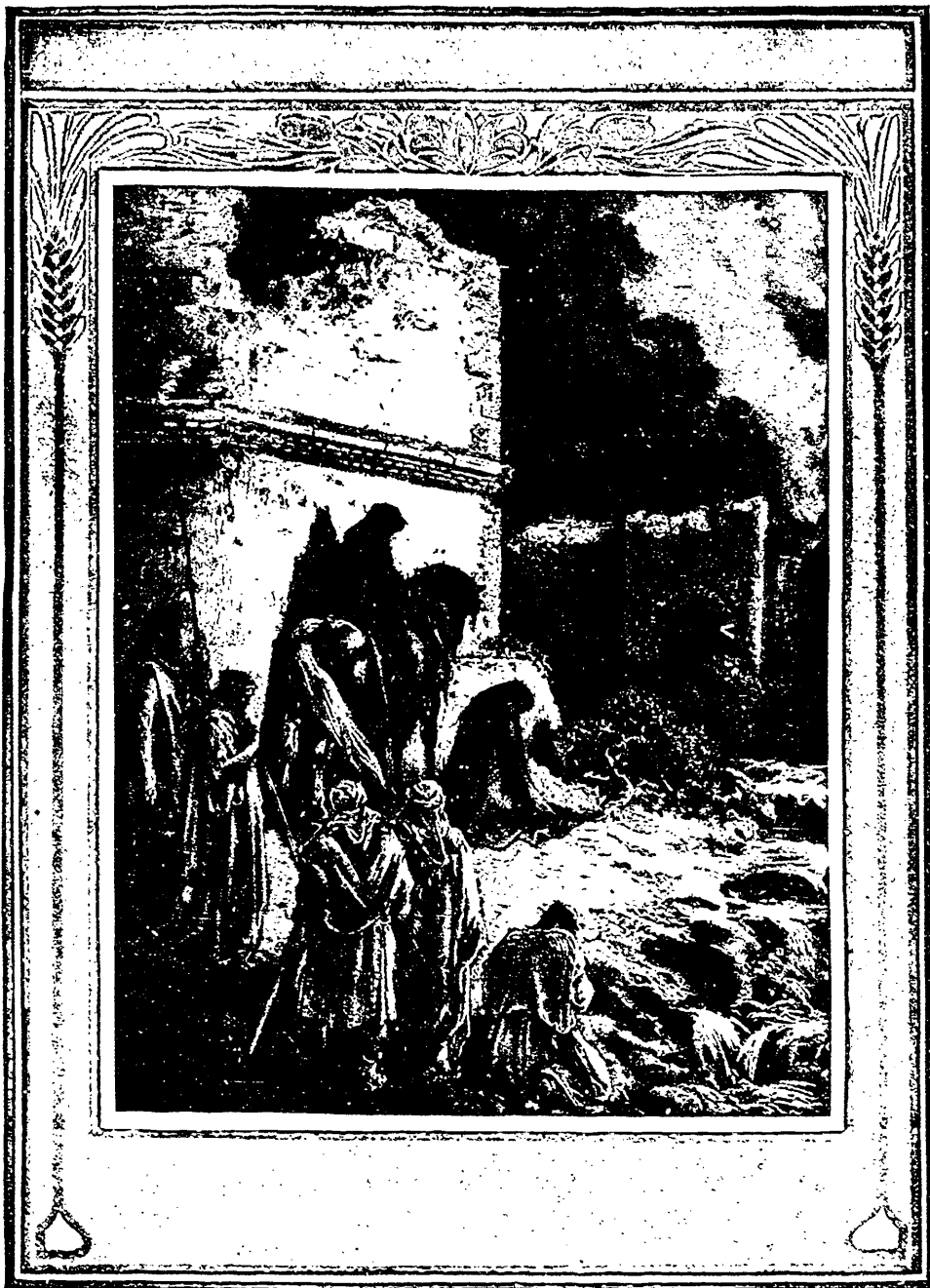
NEHEMIAH VIEWING SECRETLY THE RUINED WALLS OF JERUSALEM.
