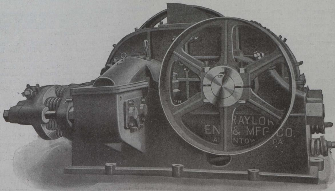
Owing to the automatic lateral shifting device, you get the maximum tonnage per set of shells and consume the minimum horse power; for all *corrugating* and *flanging* of the roll shells are eliminated by this strong, simple and positive device.
