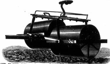
It rolls all the ground, no matter how rou There is no axie shaft, no strain, ar consequently no wear. It is easily olled between the drums,
