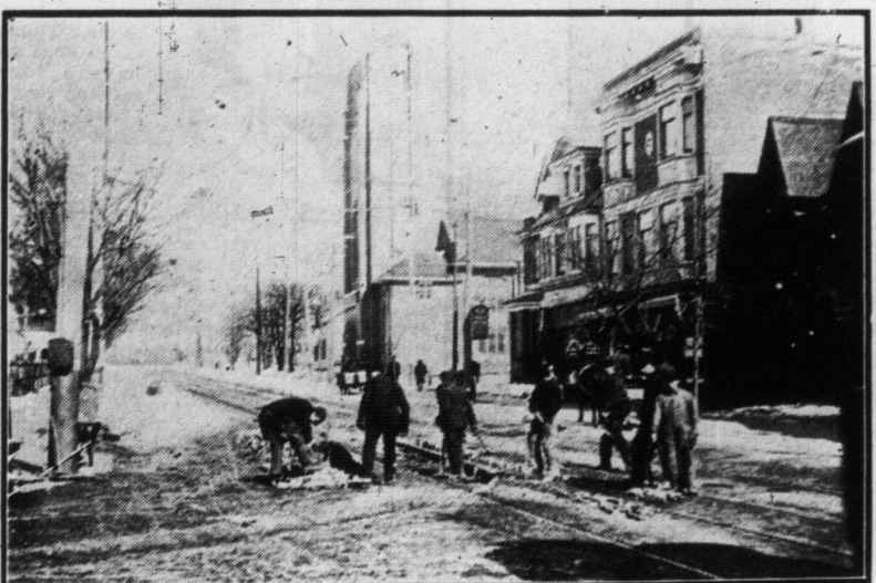
KEEPING OUR STREET RAILWAY IN ORDER. Workmen raising a bad piece of track at the corner of Broadview-avenue and Gerrard-street.
