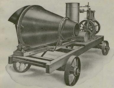
A BATCH IN THIRTY SECONDS. OUR NEW IMPROVED MIXER FOR WORK OF ANY KIND MIXES 4 TO 5 CUBIC FEET TO A BATCH.
