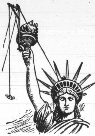
RAISING THE LAST PIECE INTO PLACE.
