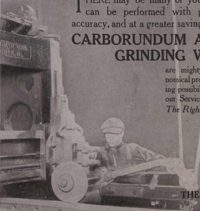
GRINDING SHEAR KNIVES ON A PLANER
