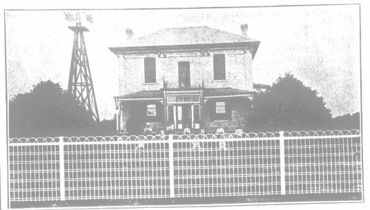
For enclosing front lawns or wherever something extra neat is wanted, our 2 in. Iron Posts with 11/4 in. Top Rail should be used, as shown in the illustration above. For ordinary purposes, neatly trimmed or fancy turned cedar posts, with a top scantling, can be used. This top rail is necessary in all cases for supporting the heavy material.
