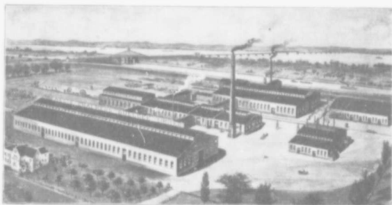
General View of ALLIS-CHALMERS BULLOCK'S Limited, WORKS, LACHINE, P.Q.
