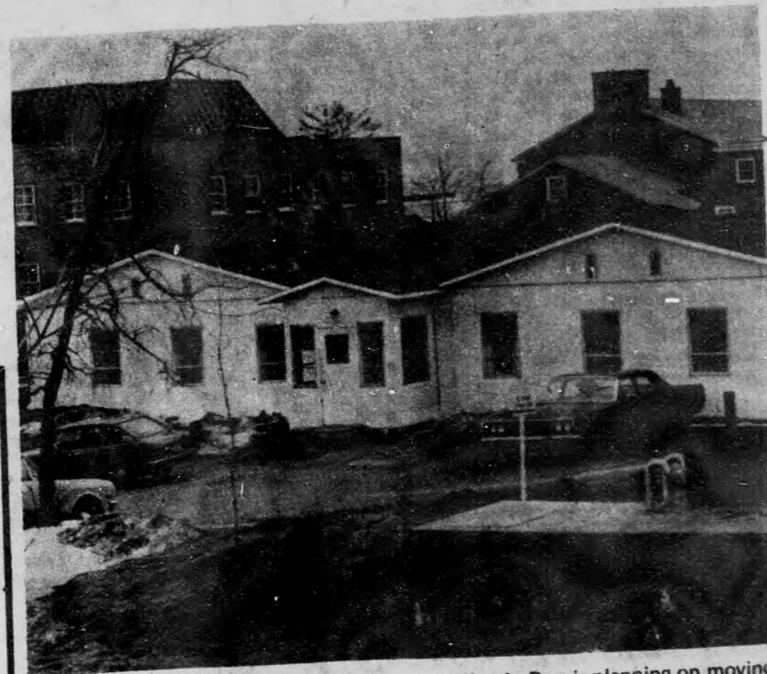
NEW RESI-DUNCE — Sorta Reeksa Crappa King LeRoy is planning on moving closer to the people by taking over Annex B as his temporary royal den.
