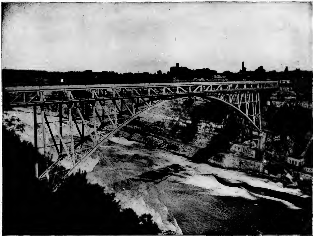
THE LOWER STEEL ARCH BRIDGE. —What is known as the Gorge is crossed at its narrowed point by an arch bridge built in 1897 by the Grand Trunk Railway. The arch is of 550 feet span, and supports two roadways, the topmost for trains, and the lower for wagons. A fine view of the Rapids may be had from this bridge.
