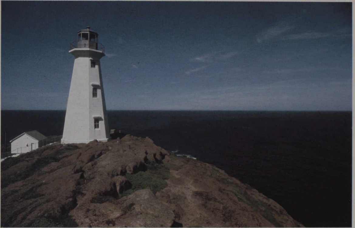
The lighthouse at Cape Spear, Newfoundland, the easternmost point in North America.
