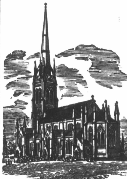
St. James' Cathedral, King St., Toronto, contains 500,000 cubic feet of space and is successfully heated with four of our Economy Heaters.
